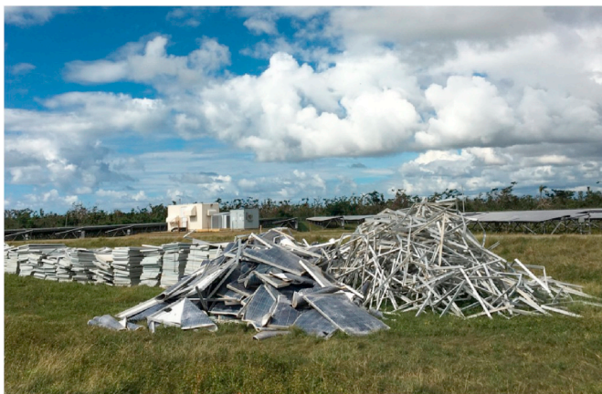
Fig. 5. Damaged panels, frames and mounts are seen at the 24-MW Illumina solar plant in Puerto Rico collected for recycling. (Source: Maria Gallucci/IEEE Spectrum).
